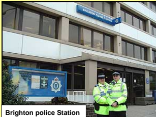
Brighton police Station
